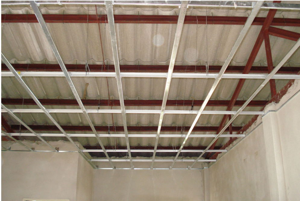
Figure 26: Steel roof framing and aluminum frame for ceiling
