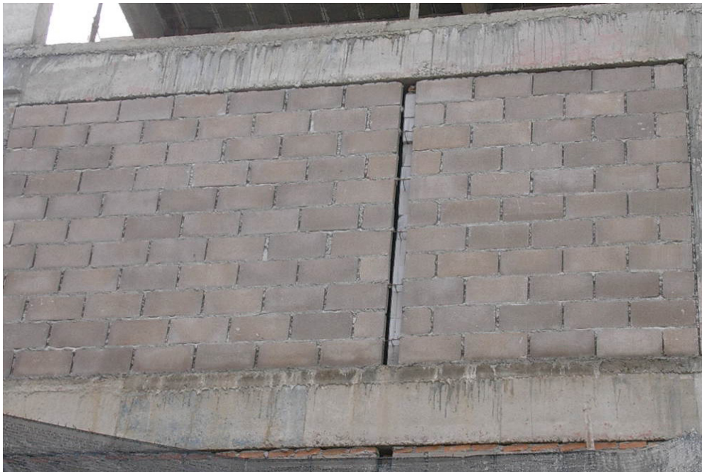
Figure 20: Concrete masonry unit or concrete block wall
