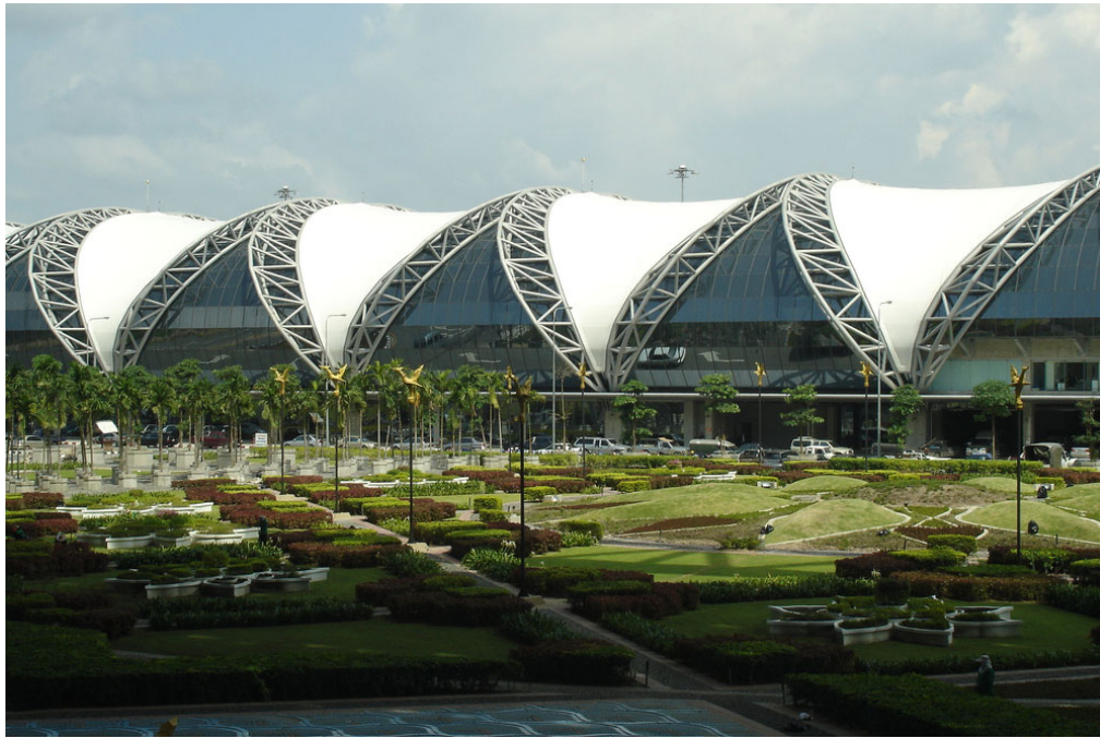
Figure 28: Glass as skylight and wall at the new Thai National Airport
