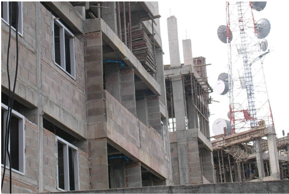
Figure 22: Concrete block construction
