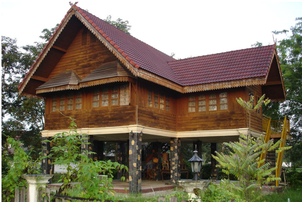
Figure 8: Contemporary Thai Northern style house where wood is still preferred.
