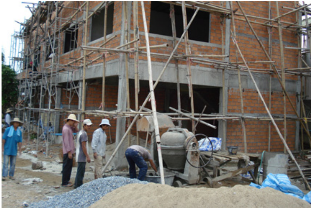
Figure 4: Thai modern architecture: construction with column and beam concrete and brick masonry wall
