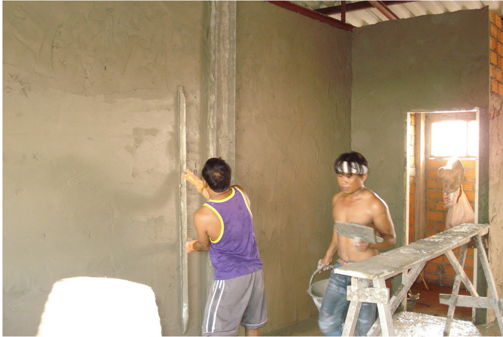
Figure 16: Masonry walls in Thailand are usually plastered
