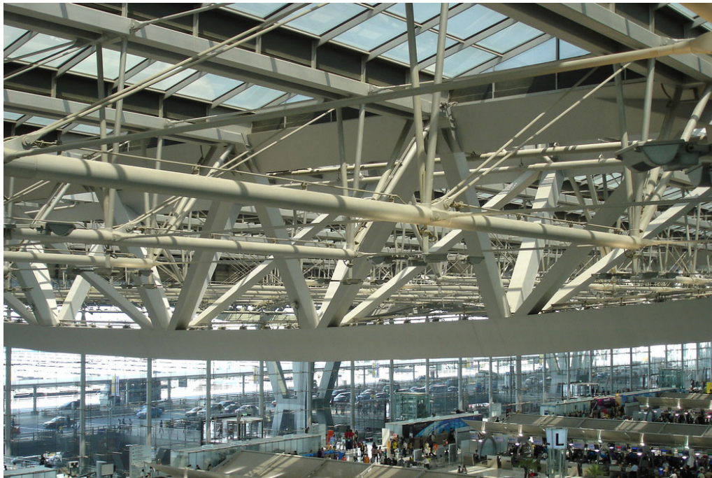
Figure 24: Steel as main structure in Thai national airport terminal building
