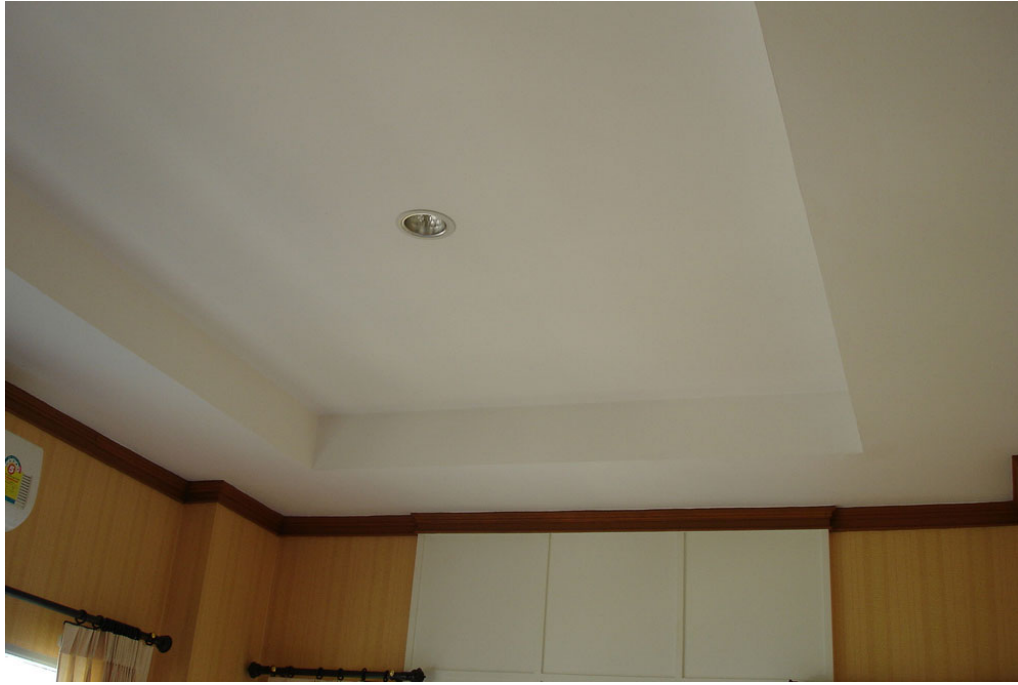
Figure 31: Seamless gypsum board ceiling can be found in high cost buildings
