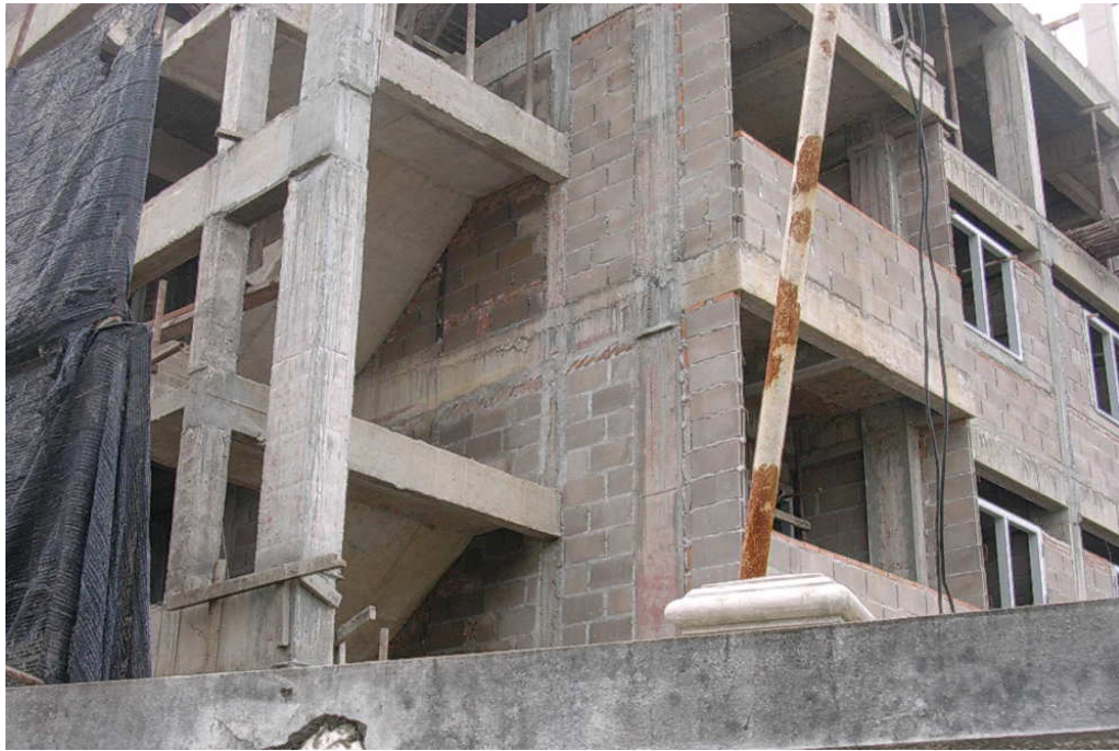
Figure 12: Concrete construction in Thailand
